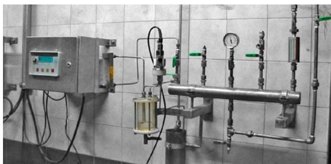
Fig. 3 CO 2 sampling for flow cell 32001 and EC sensor
